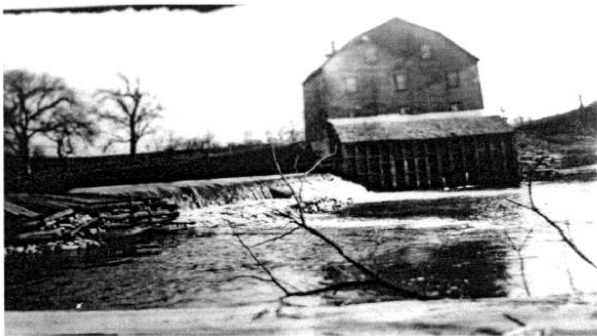
The North Mill dam, showing the back of the old mill and the lean-to built to house the flume and water wheel.
