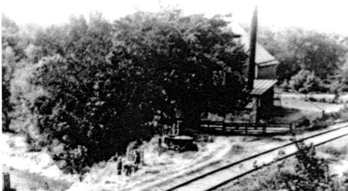
The back of the South Mill, showing the power plant added in 1893 and the south branch railroad.
