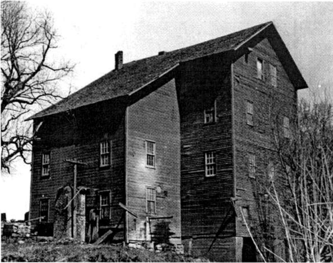
In 1893 an addition was built on the back side of the mill.
