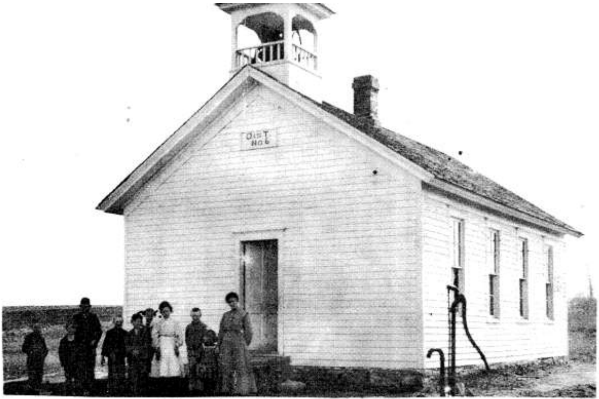
Scott Township No. 6 – Hausen (1)
