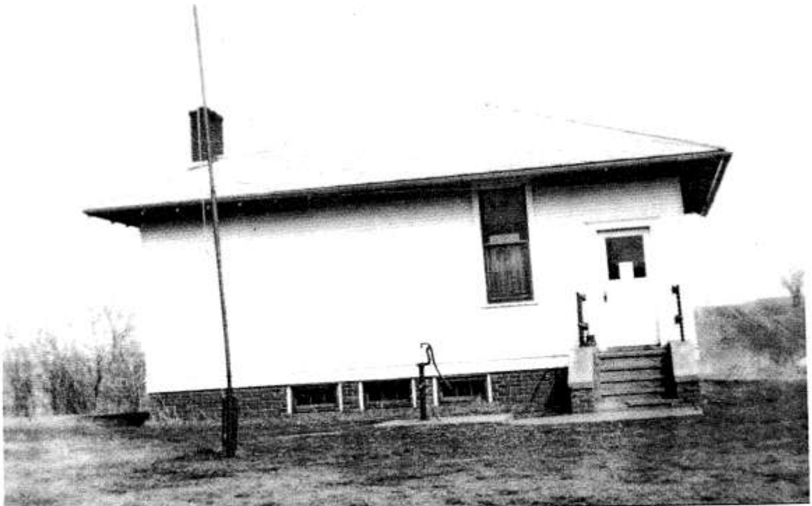
Red Oak Township No. 5 – Center, Ratliff (3)
