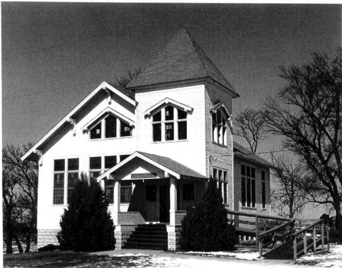
STRATTON UNITED METHODIST CHURCH, SHERMAN TOWNSHIP
